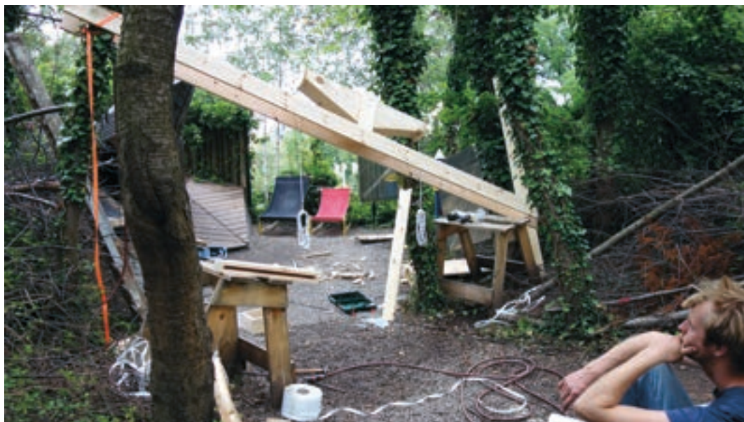
Wouters conçoit la douche du sauna / Wouters thinking up a system for the sauna shower
